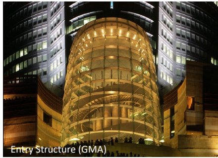
Entry Structure (GMA)
